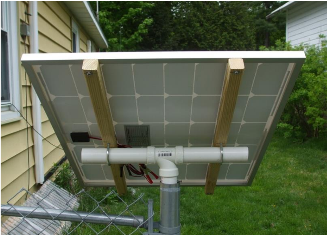
A rear view of Peter's installation, showing its genius flexibility. Note that it is mounted in a fence post to allow a wide degree of azimuth adjustment. You can just see the set screw in the PVC sitting on top of the fence post, preventing the cell from falling inside the post. Also note the U bolts holding the frame of the cell to the horizontal PVC mounting. They are used to adjust the elevation. Peter says that he rarely makes any elevation adjustments, as the solar cell works well over a wide range of settings.
